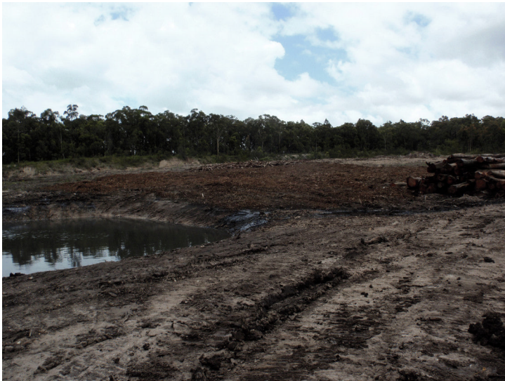
Photographic Plate Thirty Two: Clean water catchment dam and land clearing 14/12/2011
