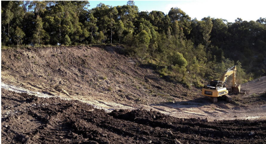
Photographic Plate Eighteen: Commencement of Southern High wall rehabilitation 2/5/2013
