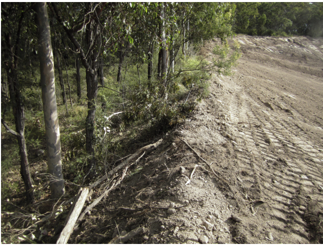
Photographic Plate Nineteen: lowering of Southern High wall bund 8/5/2013
