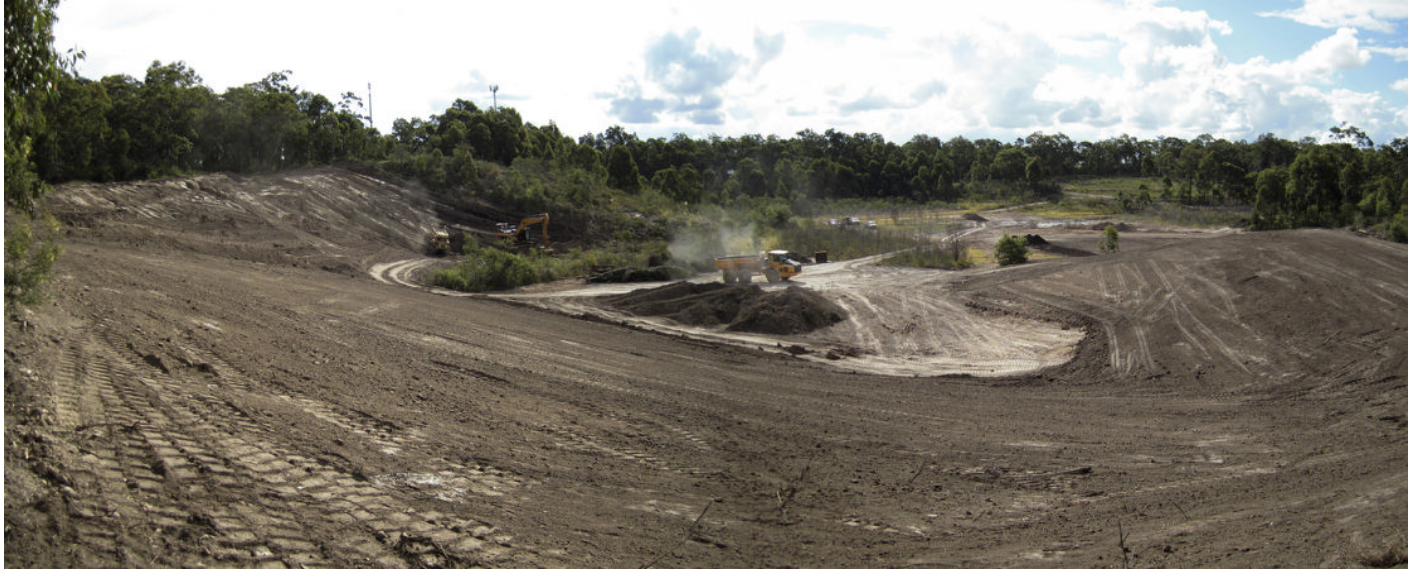
Photographic Plate Twenty: Southern High wall rehabilitation 8/05/2013
