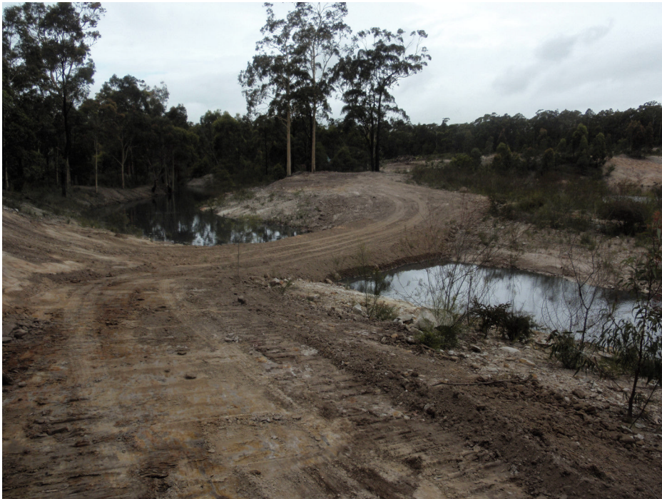
Photographic Plate Twenty Six: Central Pit and drain rehabilitation 7/12/2011
