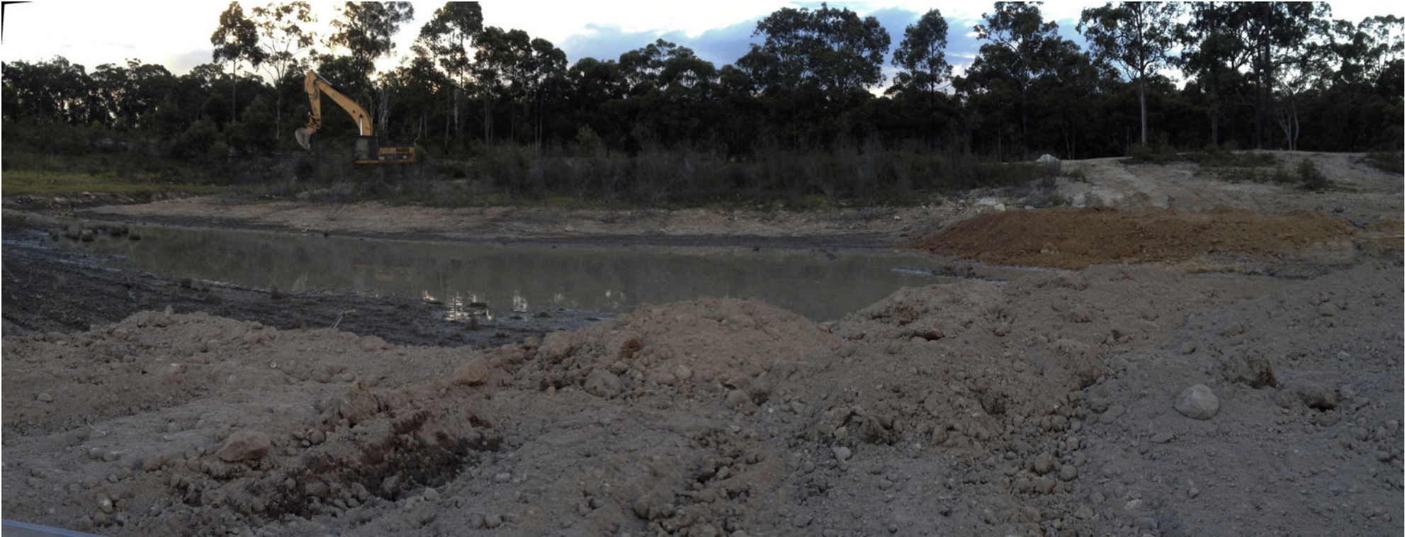
Photographic Plate Twenty Nine: Central Pit and drain rehabilitation 18/04/2013
