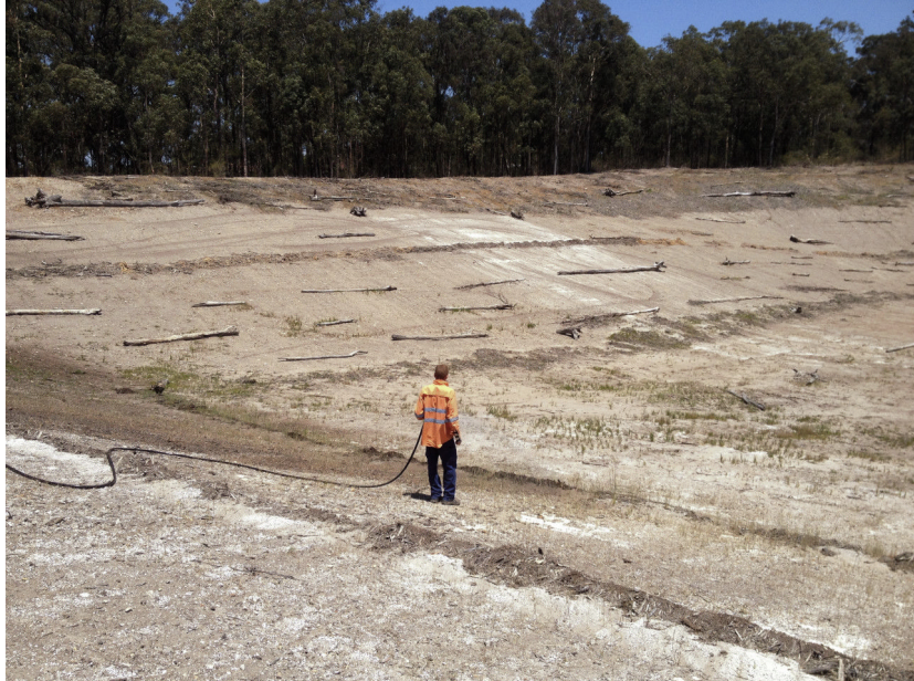
Photographic Plate Twenty Three: Southern High wall rehabilitation trials 17/11/2013
