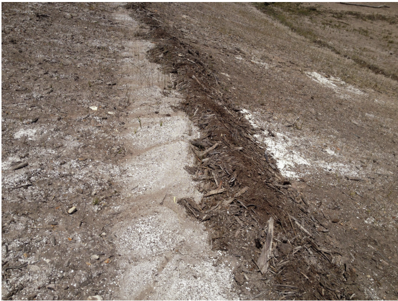
Photographic Plate Twenty Two: Mulch berms on Southern High wall 17/11/2013
