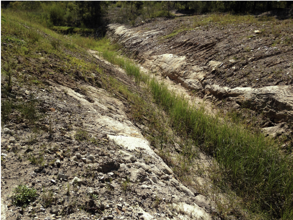
Photographic Plate Twenty Eight: Central Pit and drain rehabilitation 14/03/2014
