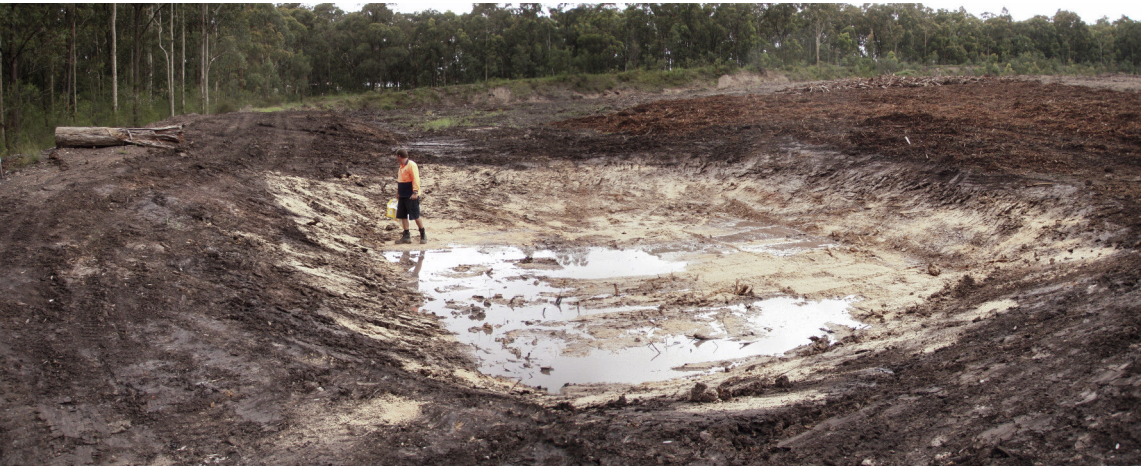
Photographic Plate Thirty: Clean water catchment dam construction 12/12/2011
