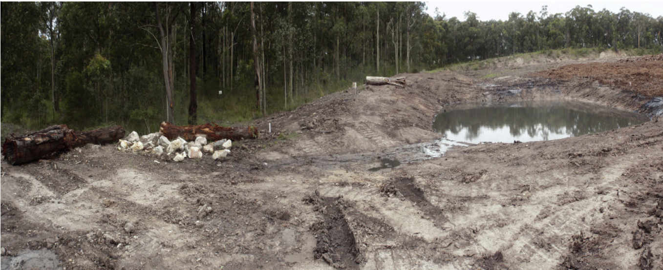
Photographic Plate Thirty One: Clean water catchment dam 14/12/2011
