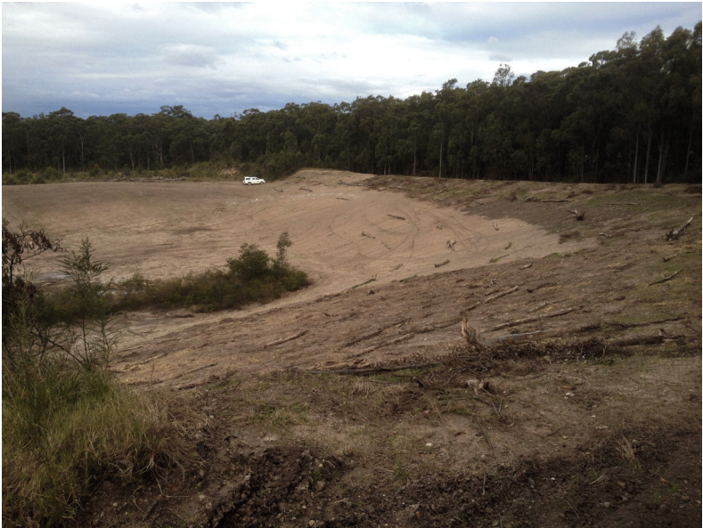
Photographic Plate Twenty One: Southern High wall rehabilitation 17/06/2013
