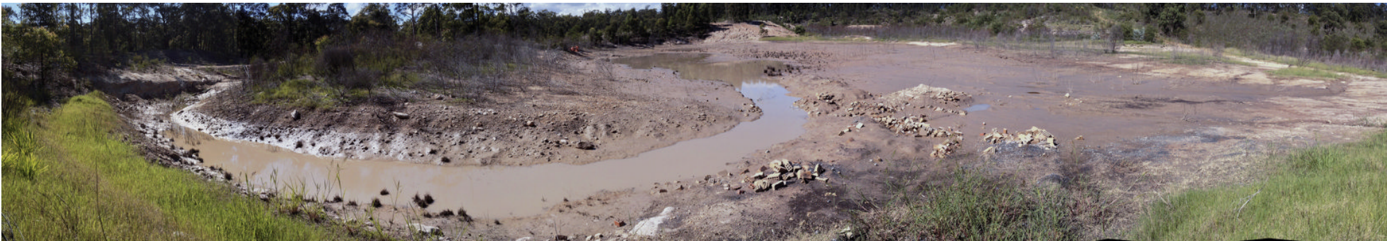
Photographic Plate Twenty Seven: Central Pit and drain rehabilitation 14/02/2013
