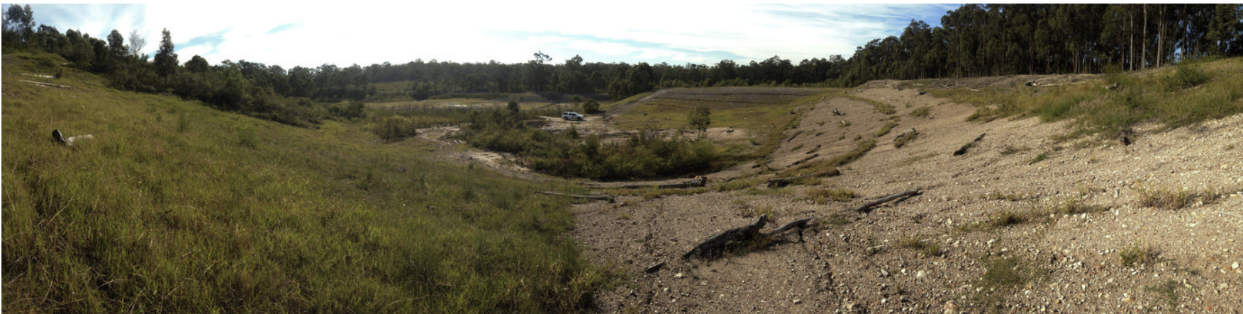
Photographic Plate Twenty Five: Southern High wall rehabilitation 14/03/2014
