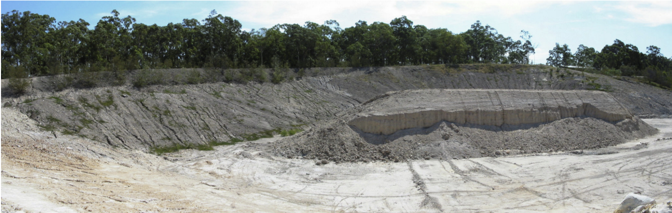
Photographic Plate Two: Southern Highwall battered back 17/1/07
