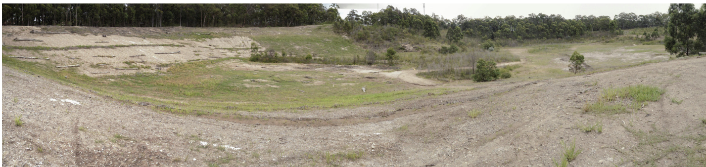
Photographic Plate Six: Southern Highwall rehabilitation progress 3/3/2014
